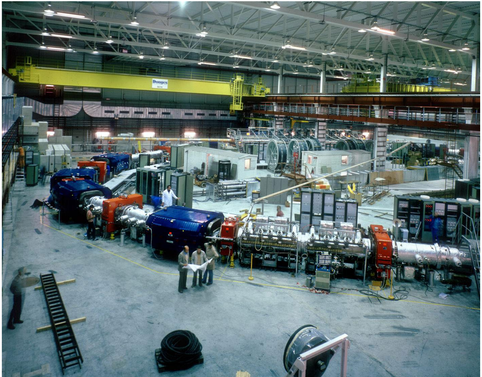
AA - a large aperture ring of different magnets - during construction.
